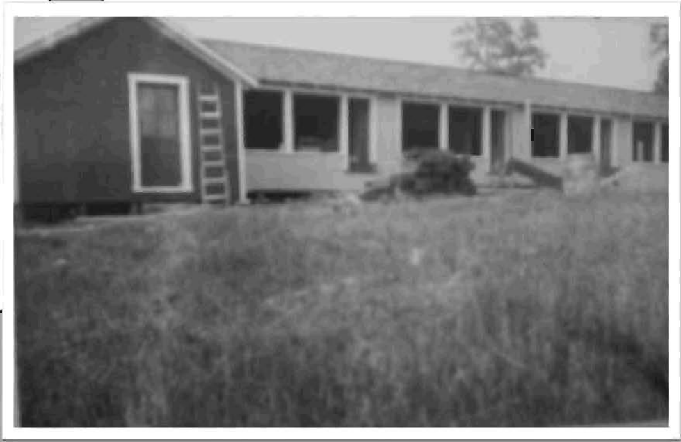
► Construction at the farm
